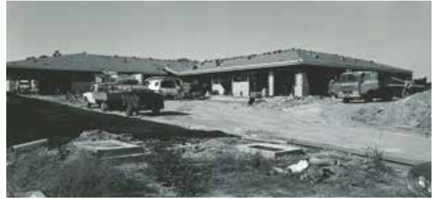
Our first home, Archbishop Duhig Court, under construction in 1978.
